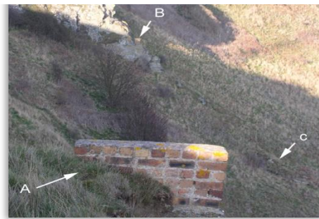
Below: the remains of a searchlight post.
